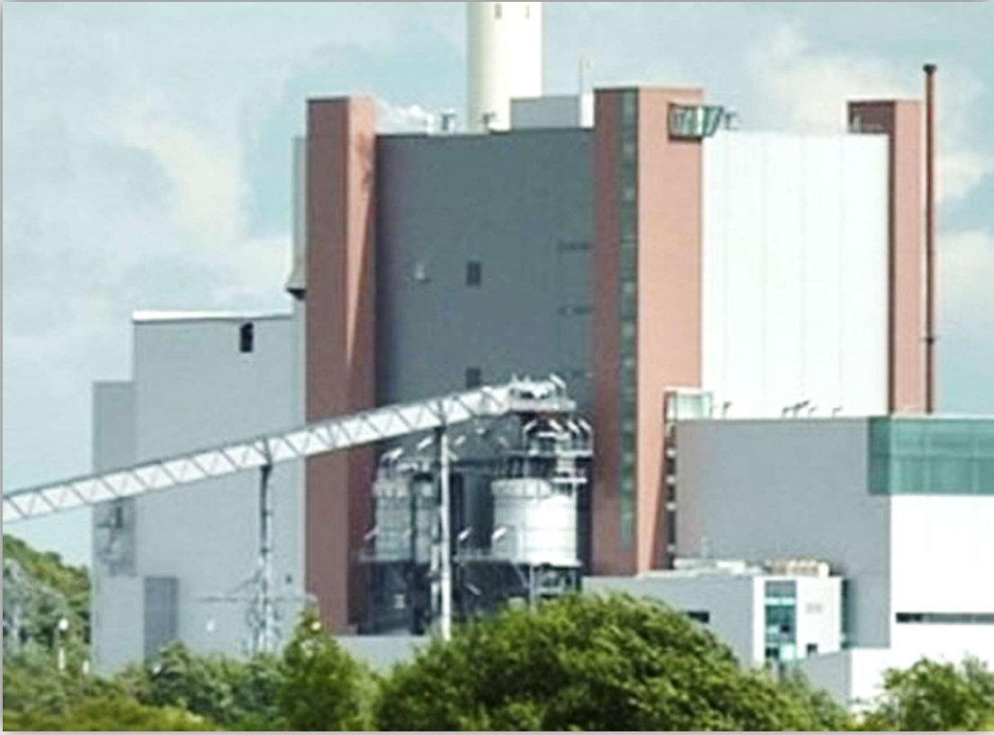
plant side view – fuel-feeding system in front of the boiler house
